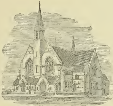
Westgate Chapel, Cleckheaton.
